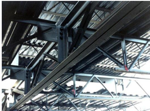
Figure 3. Flush Frame Joist-to-Joist Girder Connection
