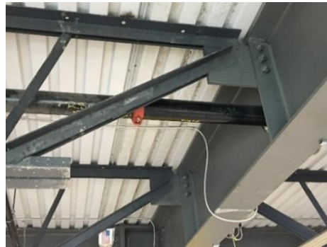
Figure 1. Typical Beam and Joist Connections to Girders
